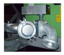
With the low pressure shut-off valve option, a shut-off valve is opened quickly at the end of the irrigation run, releasing quite a big water stream into the open. This causes a sudden pressure decrease in the supply line (to about half the original pressure). Through this drop in pressure a pressure switch shuts off the pumping unit and thus also the water supply. Therefore this valve can only be used in combination with an automatic pump shut-off device.
